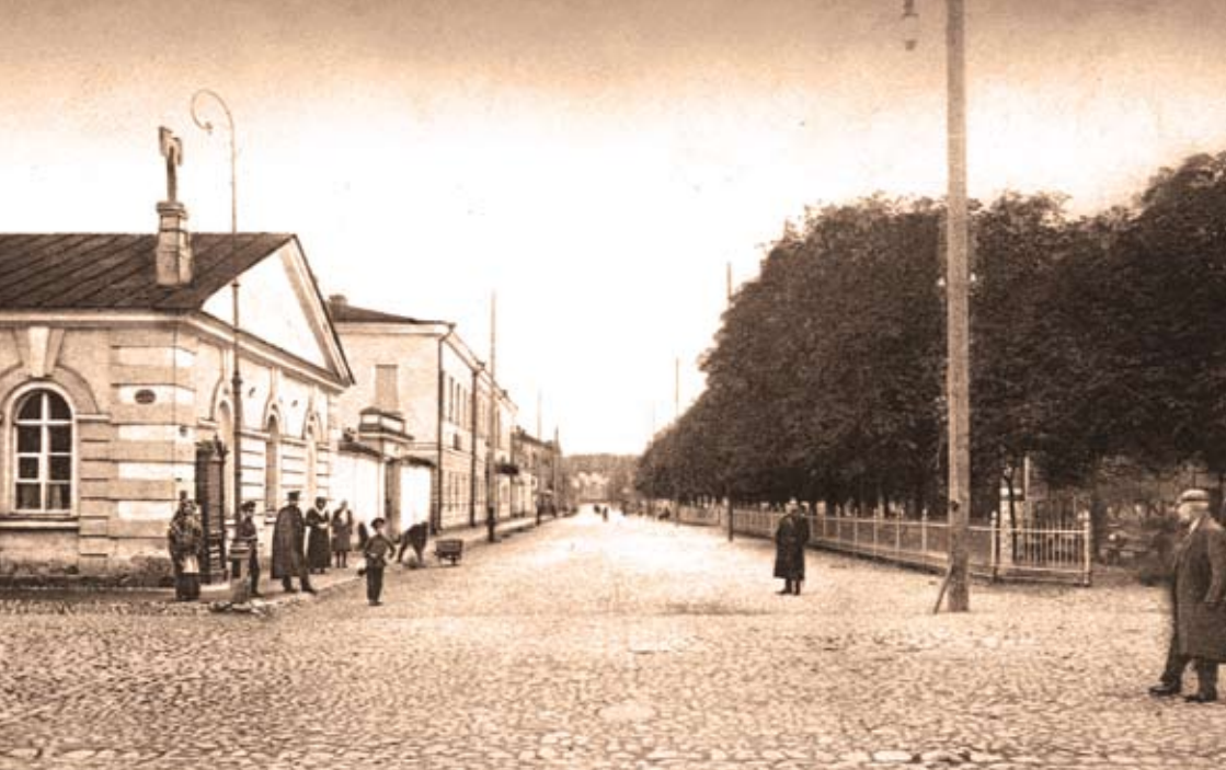
Oficieru Street (beginning of the 20th century, Lacplesa Street)
